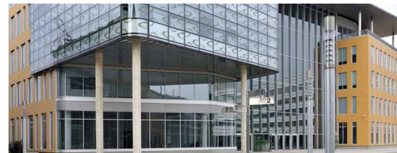
"WTC Almeda Park", Building 6, Avinguda de la Fama, Barcelona / Spain
