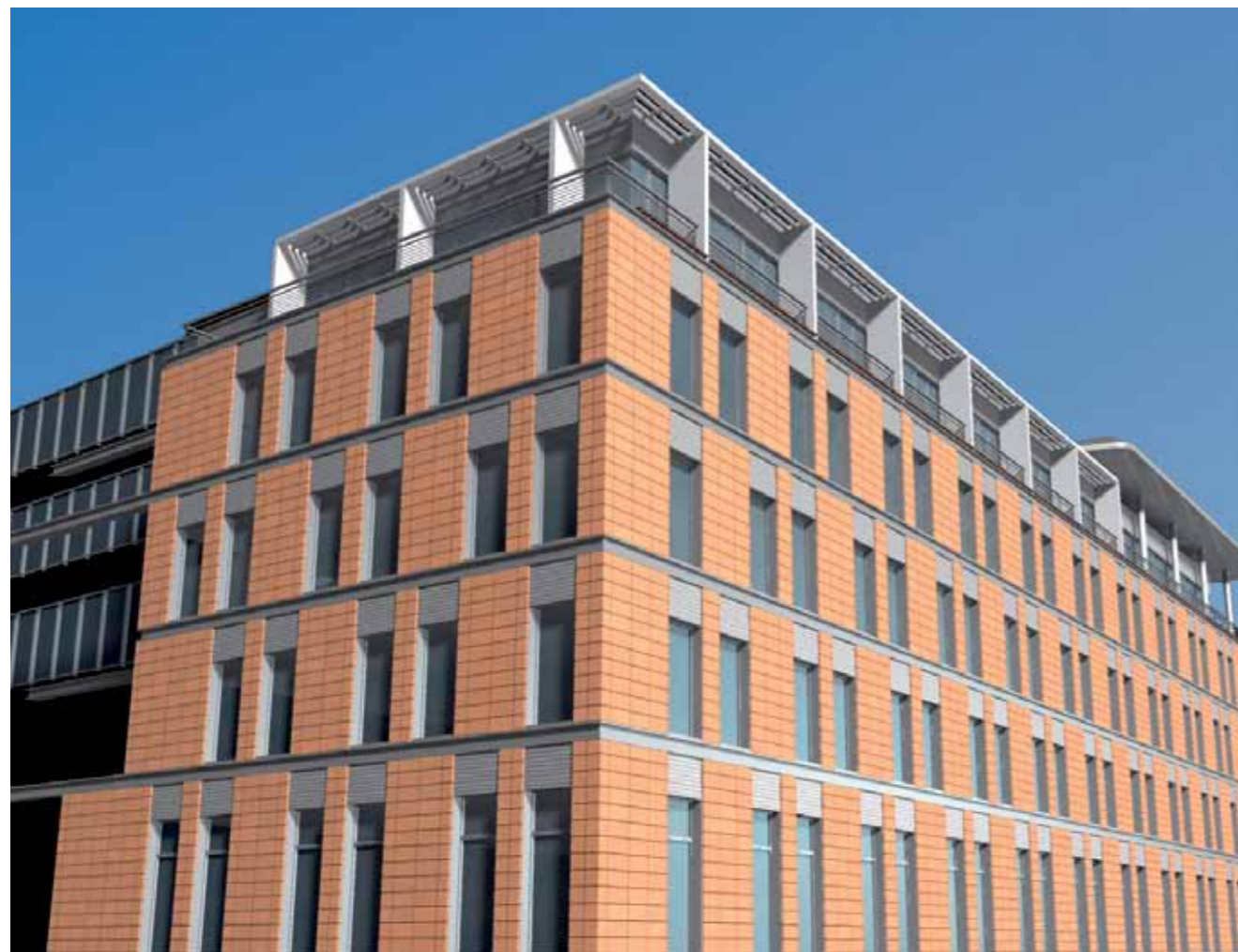
"WTC Almeda Park", Building 6, Avinguda de la Fama, Barcelona / Spain
